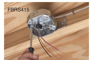
4 Install fan mounting bracket.
