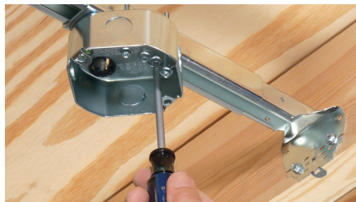
3 Adjust box position from 16" to 24" on center between joists.
