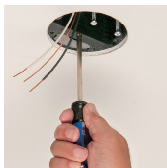
Depth adjustment screw
