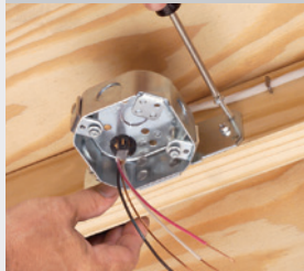
FBS415S/FBS420S Mount on SIDE of Joist
