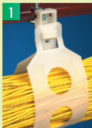
1) Single LOOP mounted parallel to beam.
