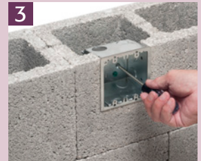
3 Tighten the screws on the spring clip to pull it securely against the block.
