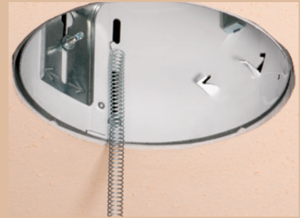
Installation Method B, No tabs inside the can or too close to fixture. Attach the springs directly to the 'can'.
