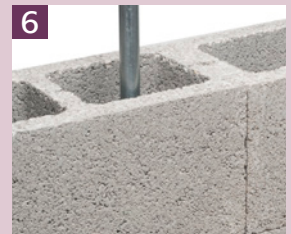
3 Tighten the screws on the spring clip to pull it securely against the block.
