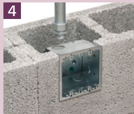
4 Install the EMT in the top of the box. Top view: EMT installed in box.
