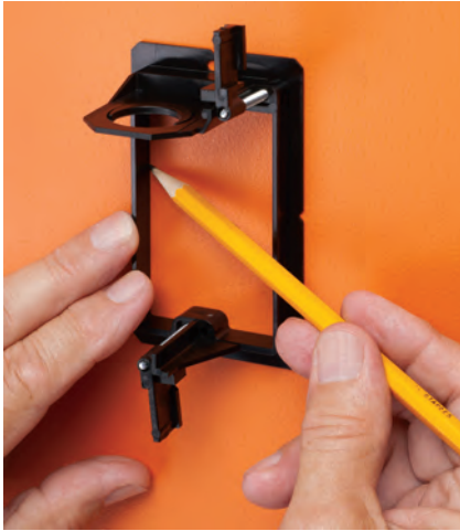
Determine bracket position. Trace along the inside of LVK1. Cut on the outside of the line.
