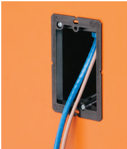
Pull low voltage wires.
