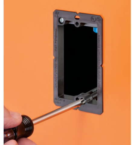
Tighten mounting wing screws.
